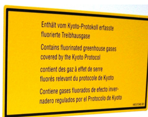
Figures 4-8 and 4-9: Additional multilingual labels are placed near the servicing access of switchgear <52 kV (left) and >52 kV (right).
